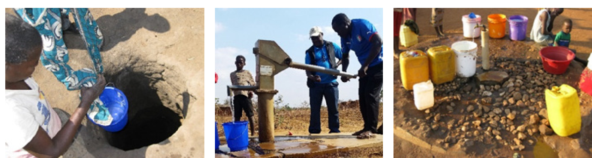
Figure 1 Sources of water in rural Malawi. Left: shallow well; Centre: hand pumped borehole with Afridev pump; Right: tap stand.
